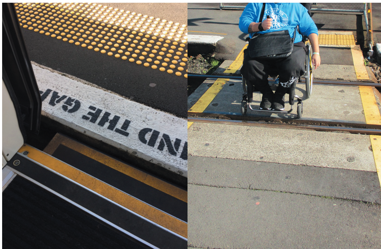
Figure 3. The gap between the train and Glen Innes station (left) and the train tracks that threaten wheelchair stability.
